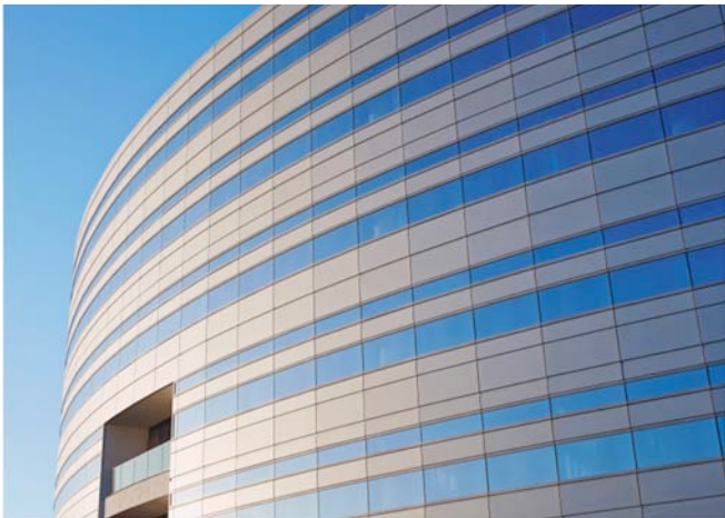
Photograph 2: Insulated Metal Panel System II —Completed building with both insulated metal panels and glazing installed.
